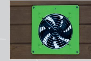
3. From the outside, install the fan cover onto the fan unit, and screw it tight, using the fastening screws provided.
